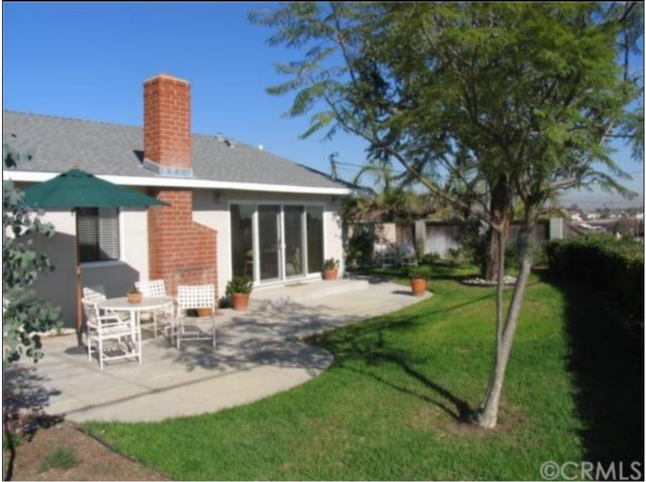
Photo 1A: 5608 White Ct before remodel.
