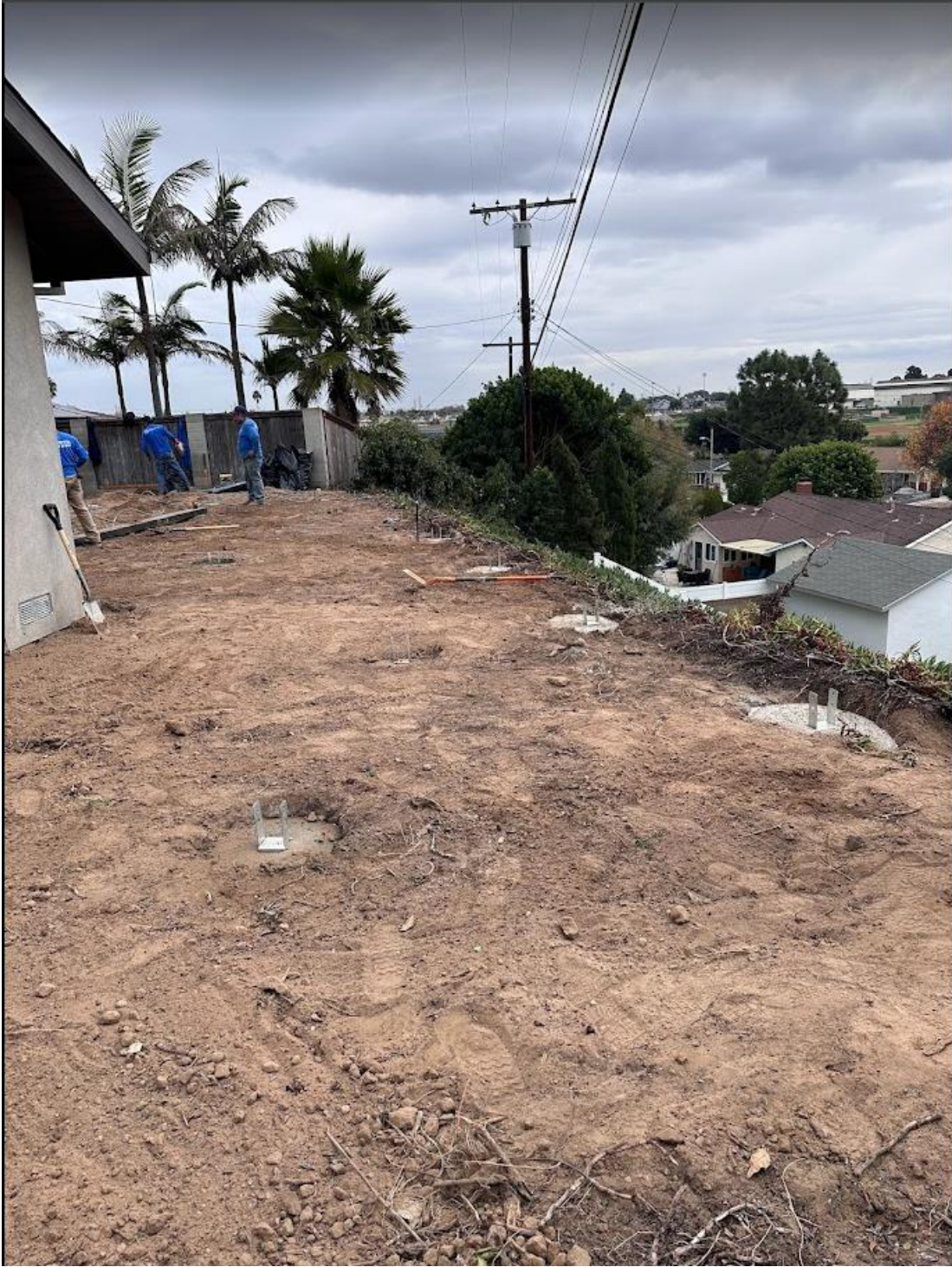
Photo 1C: 5608 White Ct during deck construction.
