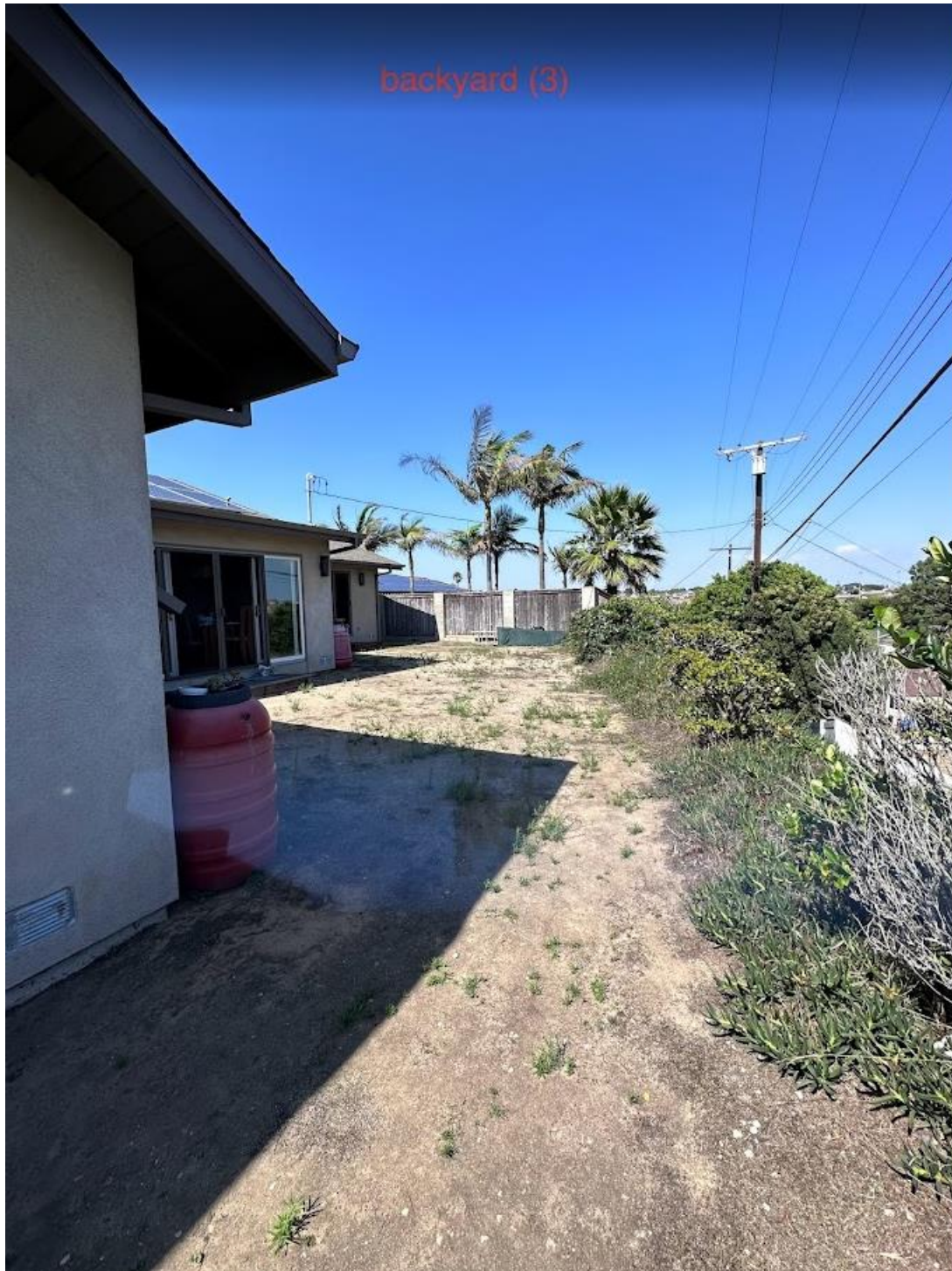
Photo 1B: 5608 White Ct after remodel before deck construction.
