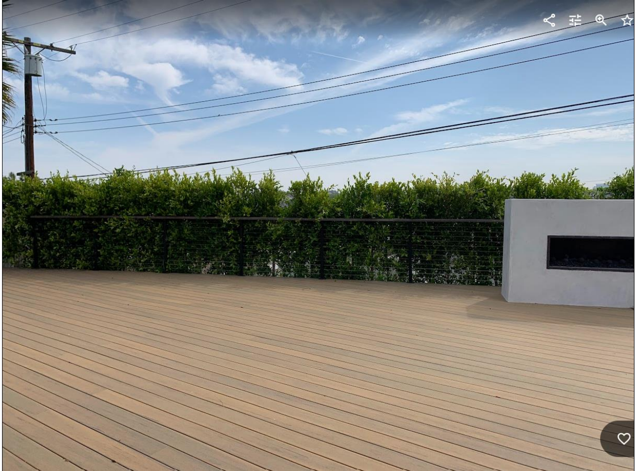
Photo 3C: 5608 White Ct before deck construction. Note: area greater than 10' and not part of 10' setback.
