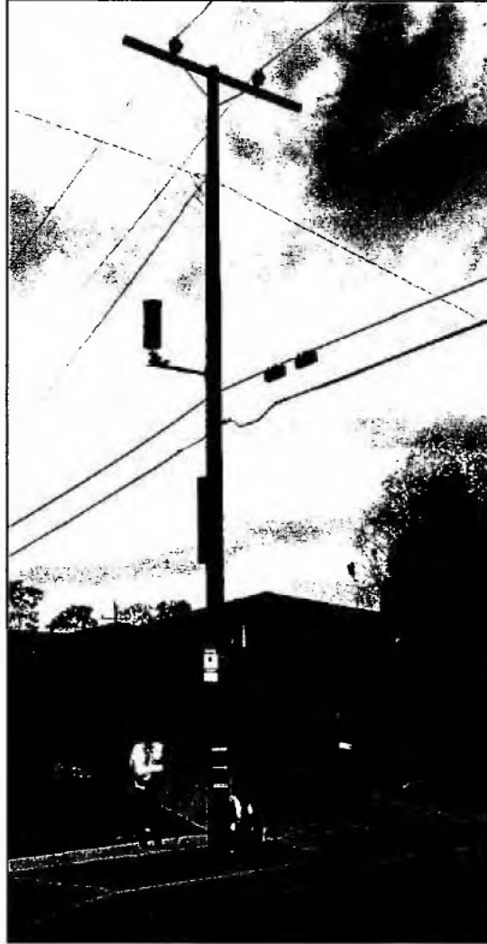
Figure 1: Omni-directional antenna, Antenna Arm, Fiber Node, 4 DC power converters, 4 RRUs enclosed within two enclosures, RF signage (e.g., connecting wires, PVC conduits, etc.) (Source: Photo Simulations provided by Applicant).
