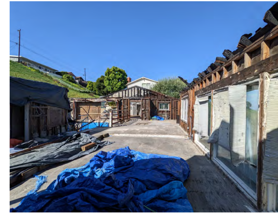
UPPER LEVEL INTERIOR VIEW
