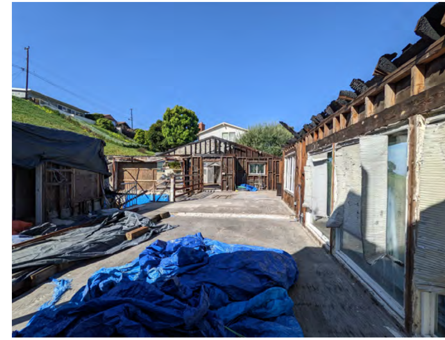
UPPER LEVEL INTERIOR VIEW
