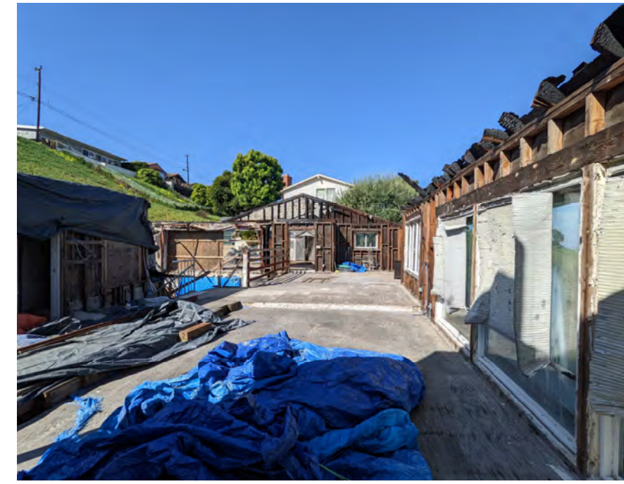
UPPER LEVEL INTERIOR VIEW
