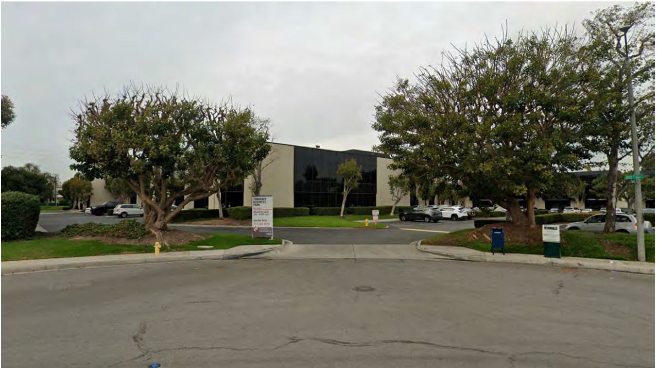
Driveway at Beech Ave and 205th St.
