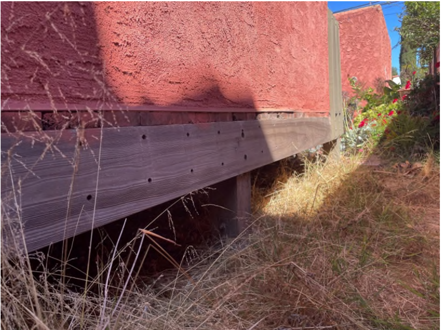
Rear room addition foundation
