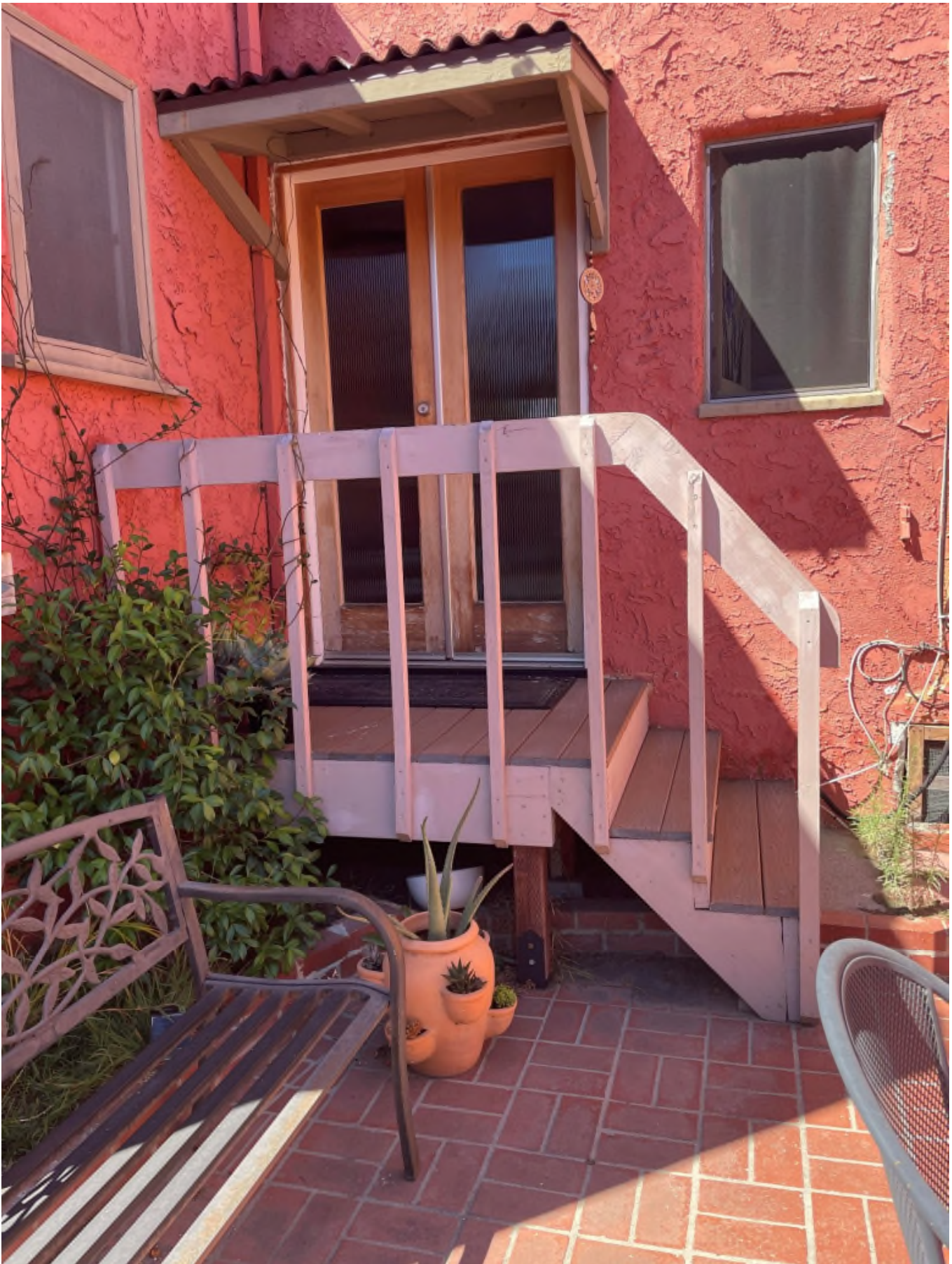
Double doors, stairs and railing to rear yard
