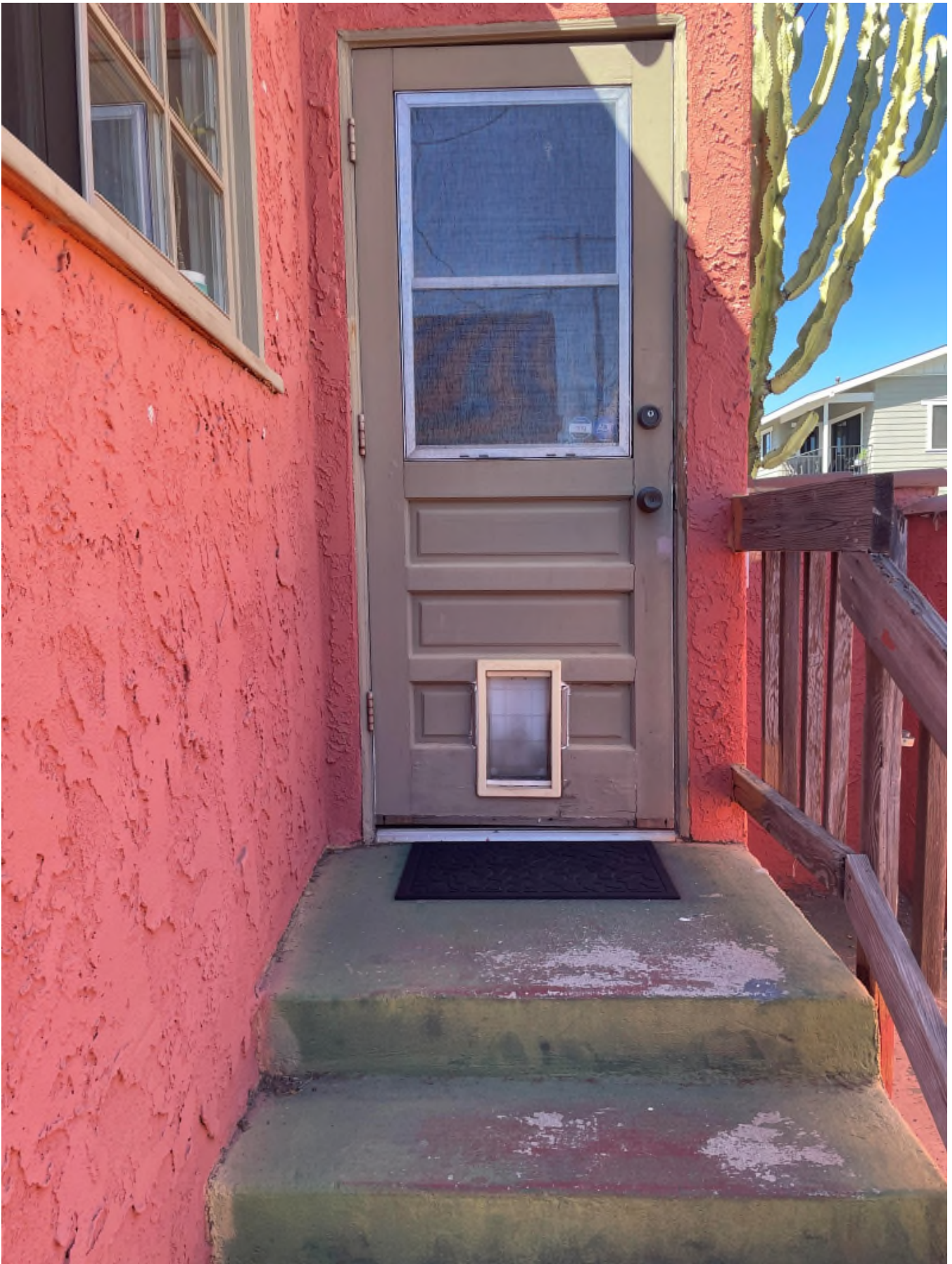
Rear kitchen door
